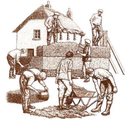
Traditional method of cob construction showing mixing, placing material on the wall, compaction by treading and paring back the wall face.
