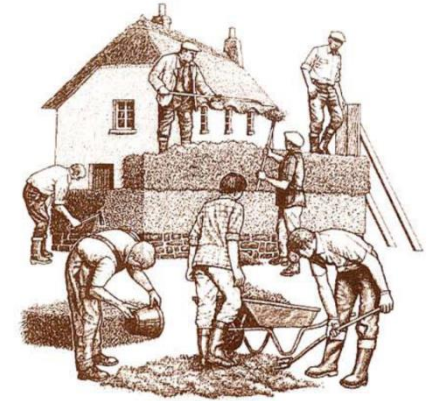
Traditional method of cob construction showing mixing, placing material on the wall, compaction by treading and paring back the wall face.
