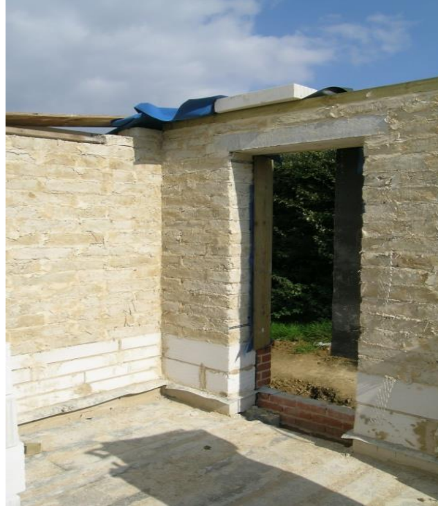
Modern earth block home under construction
