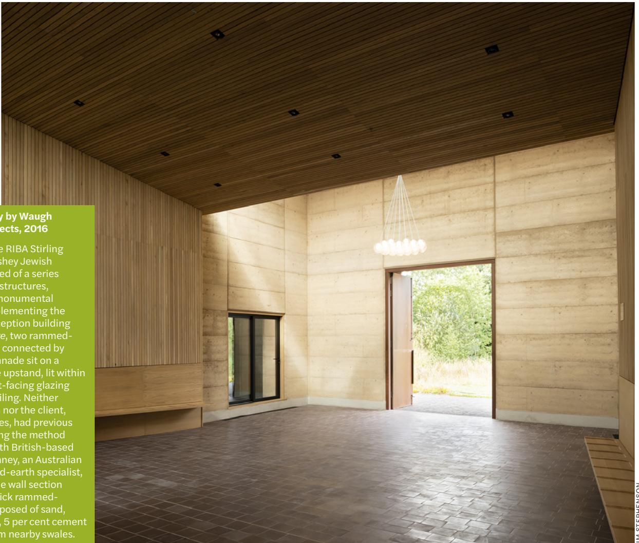
blockwork and the constituent materials are almost identical. As a result, the thermal performance is comparable. However, using earth construction could easily reduce the carbon footprint of a wall by two thirds.
