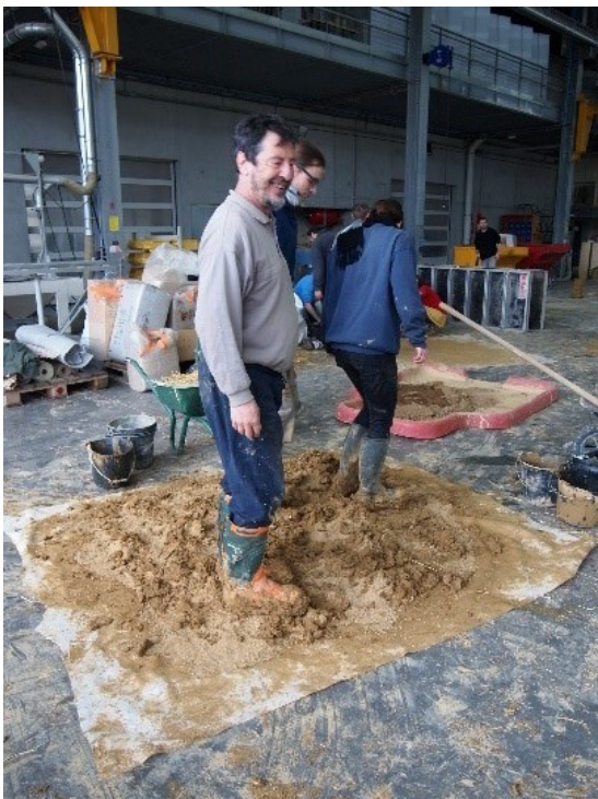
Mixing by foot on a tarpaulin, cob training, april 2018, Les Grands Ateliers de L'Isle d'Abeau
