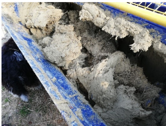
Mixing soil and flax straw with Warzee mixing bucket
