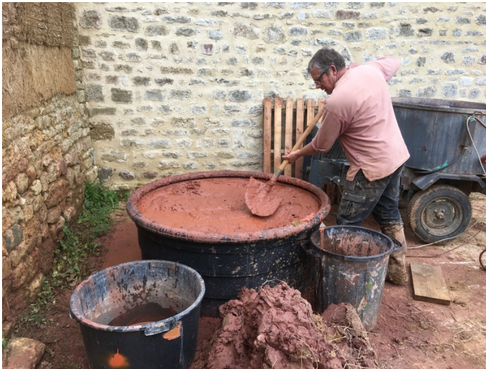
Figure 18. Mixing water with soil to form slip (Photo: François Streiff)
