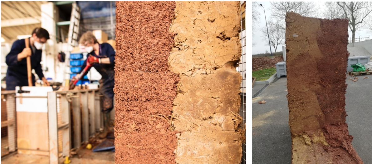
Figure 5 Photo showing angled batt / toothed joint between thermal and structural layers. (Photo: Lloyd Russell)
