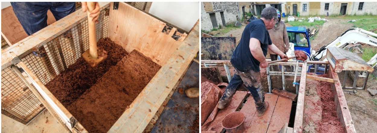
Figure 9. Photo showing filling of thermal cob layer against structural cob layer. (Photo: François Streiff)
