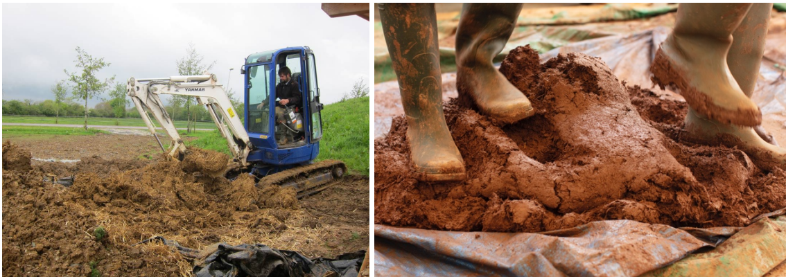
Figure 17. Mixing structural / traditional cob by machine or foot (Photo: François Streiff)
