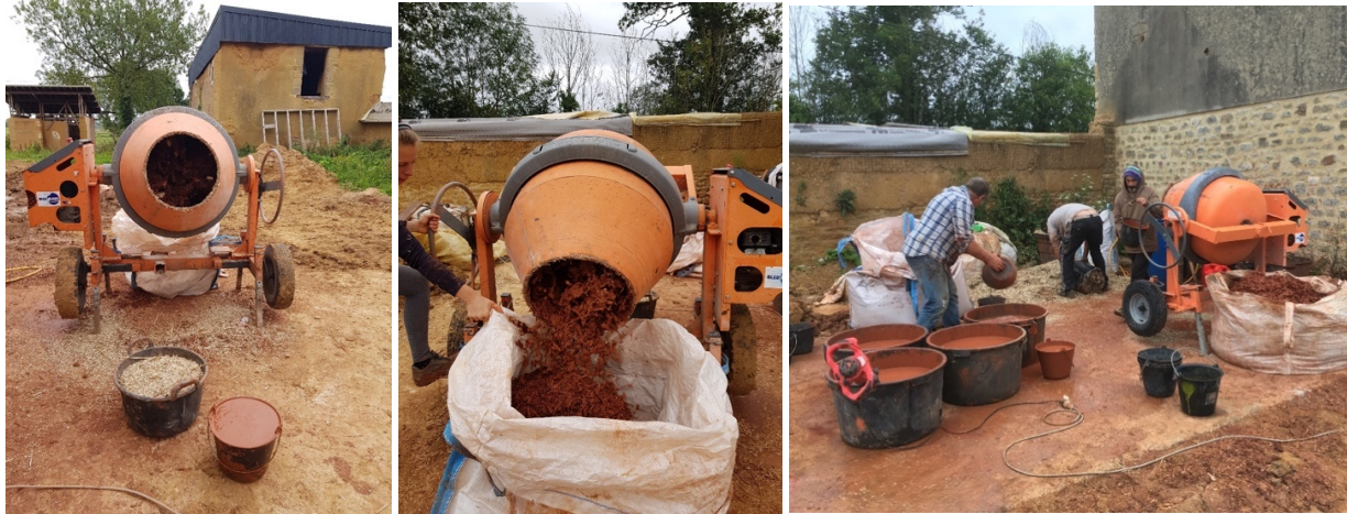
Figure 23. Photos showing mixing of thermal cob on site (Photo: François Streiff)
