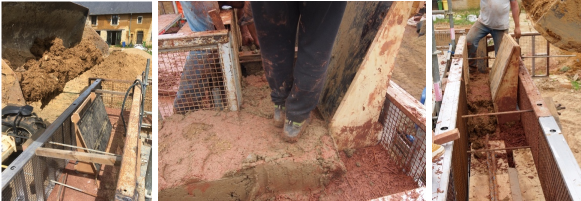
Figure 8. Photos showing the placement tool on site. (Photo: François Streiff)
