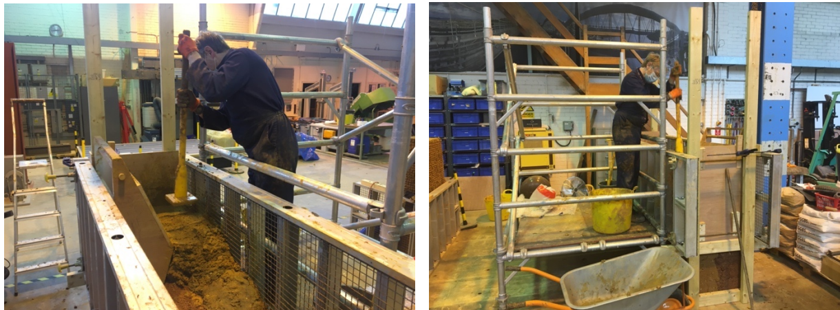
Figure 15. Photos showing the use of a small scaffold tower to aid low level construction. (Photo: Matthew Fox)
