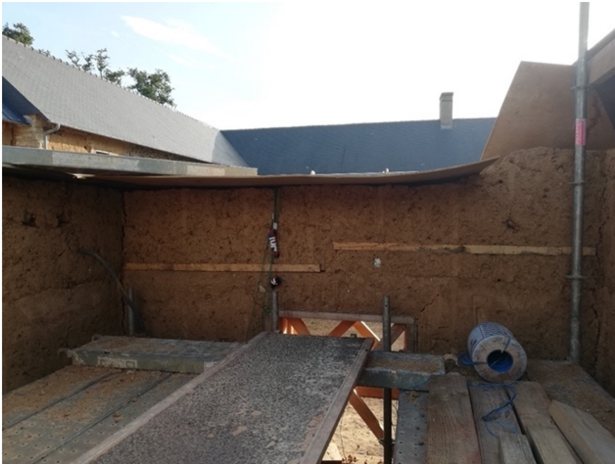
Figure 13. Photo showing sheets of timber protecting tops of wall. (Photo: François Streiff)
