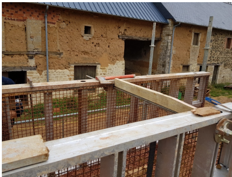
Figure 4. Photo showing spacing of formwork using wooden spacing block (Photo: François Streiff)
