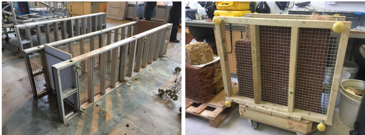
Figure 1. Photos showing metal (left) and timber (right) formwork examples. (Photo: Matthew Fox)
