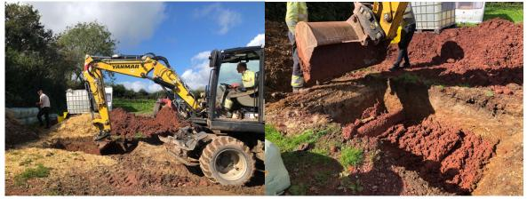
The first stage is A1 - raw material extraction and processing. Pictured above is the Yanmar wheeled excavator digging out the clay sub-soil ready for mixing.
